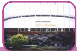
Sarawak Outdoor Stadium
