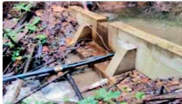
Figure 19: Mini microhydro for water supply at Rh. Manggat
